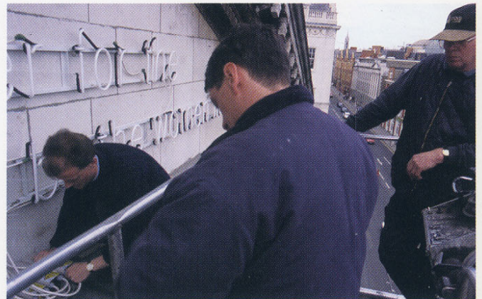
above: Installation crew, City Hall (see front cover)
